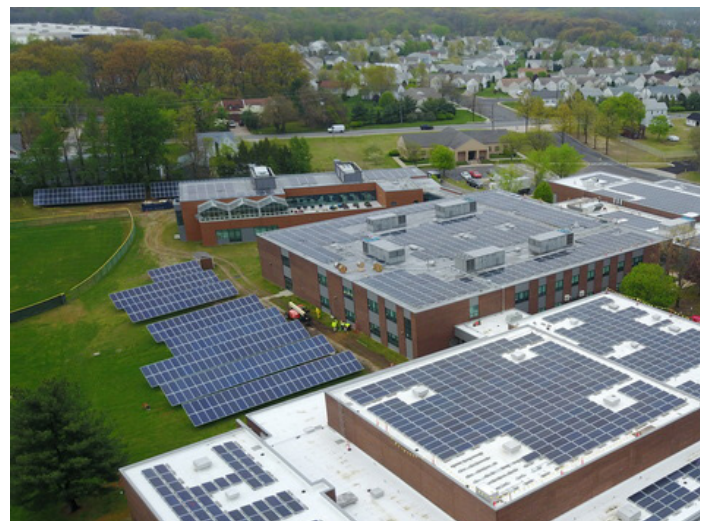
Figure 1 Delran, NJ - AEP OnSite Partners (Roof and Ground Mounted - 850kW-DC)
