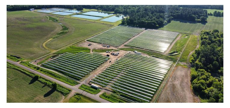
The Barron solar array is a 3.6 MW-DC photovoltaic solar generation facility located in Barron, Wisconsin. It features almost 9,000 tracking solar panels and will provide on-site renewable energy to cover a portion of the City of Barron's energy consumption for the next 30-years. AEP OnSite Partners built, owns, and operates this solar array.
